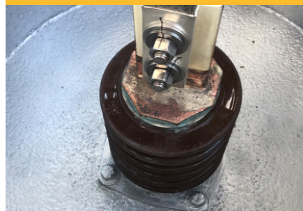
SOLUTION: CRYOGENIC CLEANING
