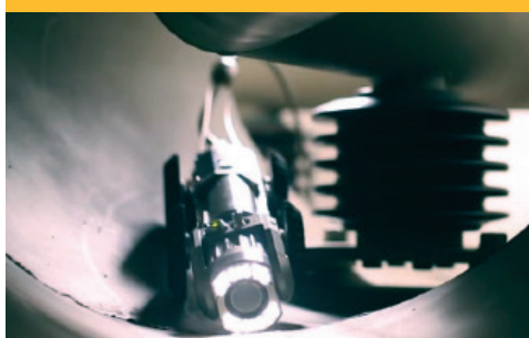
SOLUTION: ROBOTIC INSPECTION
