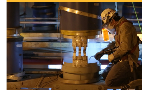
SOLUTION: CRYOGENIC CLEANING
