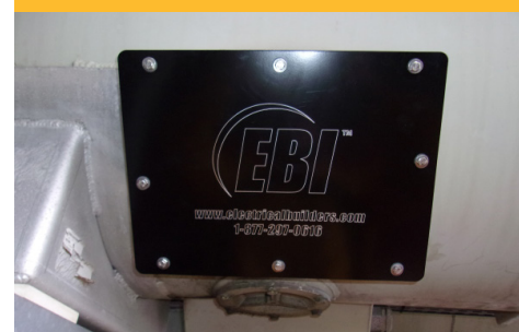
SOLUTION: WELDED INSPECTION WINDOWS
