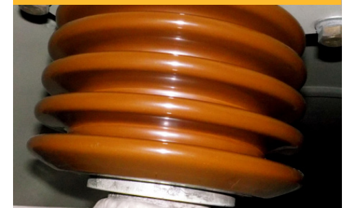
SOLUTION: CRYOGENIC CLEANING
